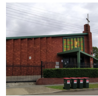
St Dominic's Church (聖道明教堂) The Crescent & Hornsey Rd, Homebush West, NSW 2140
